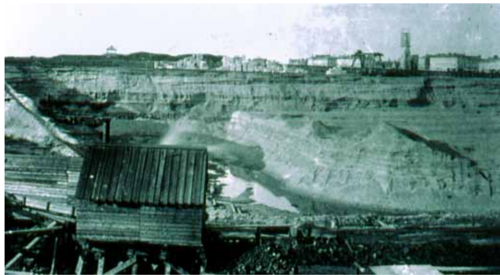
New Dock excavations. Note in the background, the seafront pagoda (Still in existence) and Christ Church steeple under construction. The pines haven't been planted yet!
