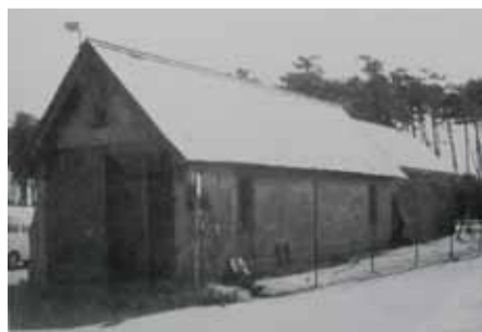
Silloth Lifeboat House with garage extension (1980 modification)
