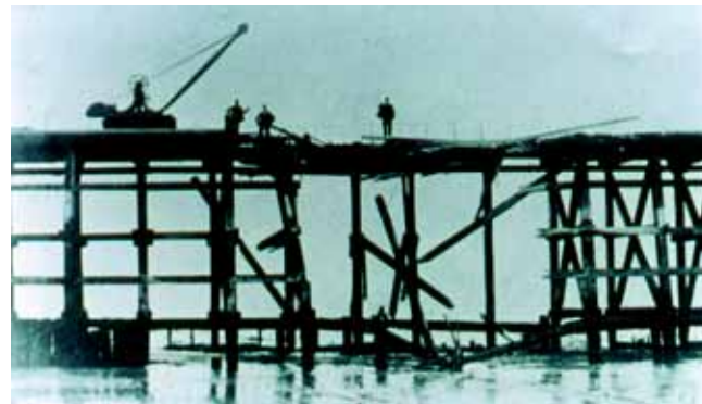
Silloth Pier damaged by shipping
