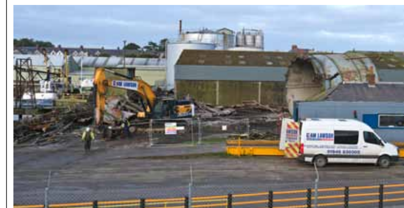
After sitting unused for over thirty years the three massive silos at Silloth Dock have finally been removed by DA Harrison.
